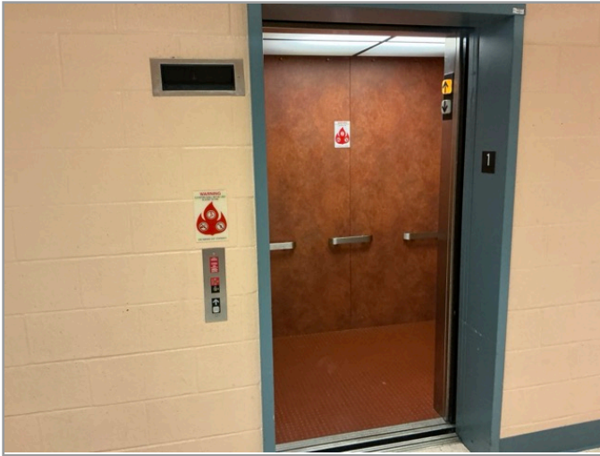
LOBBY LOOKING AT CABS
