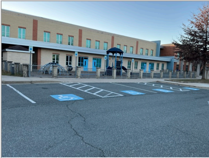
OVERVIEW OF ACCESSIBLE PARKING AREA
